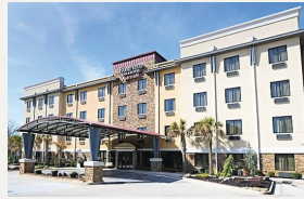
Fairfield Inn & Suites 678-971-4670
